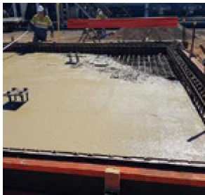
Complete Design and construction of a slurry drainage slab and sump.
