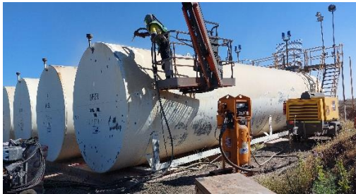
Blasting and painting of existing fuel farm tanks.
