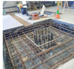
Insitu slab for crane jib incorporated into an existing structure.
