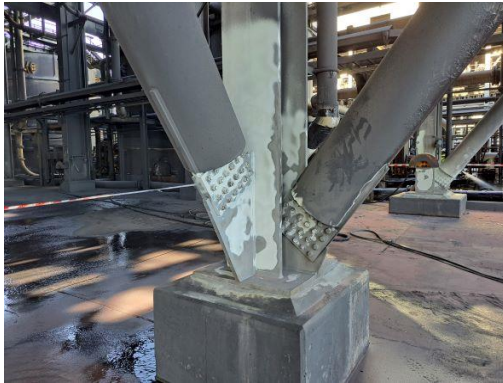
Blasting of existing steel structures in brownfields environments
