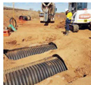
Repair of collapsed culvert section.
