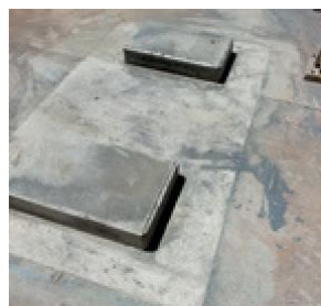
Completed concrete plinths.
