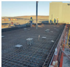
Complex reinforcement with precise drainage falls to concrete.
