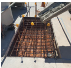
Removal of existing concrete and installation of concrete plinths.
