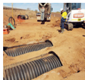
Repair of collapsed culvert section.
