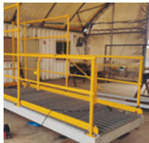
Design and site fabrication of permanent platform to replace scaffolding.
