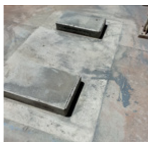
Completed concrete plinths.
