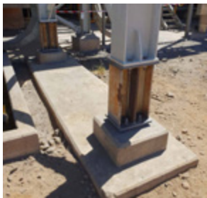
Column extensions required to lift an existing structure. Extensions designed and fabricated on site.
